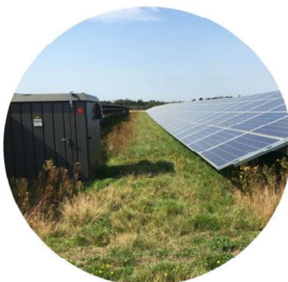
Transformerstation imellem solcellerne
